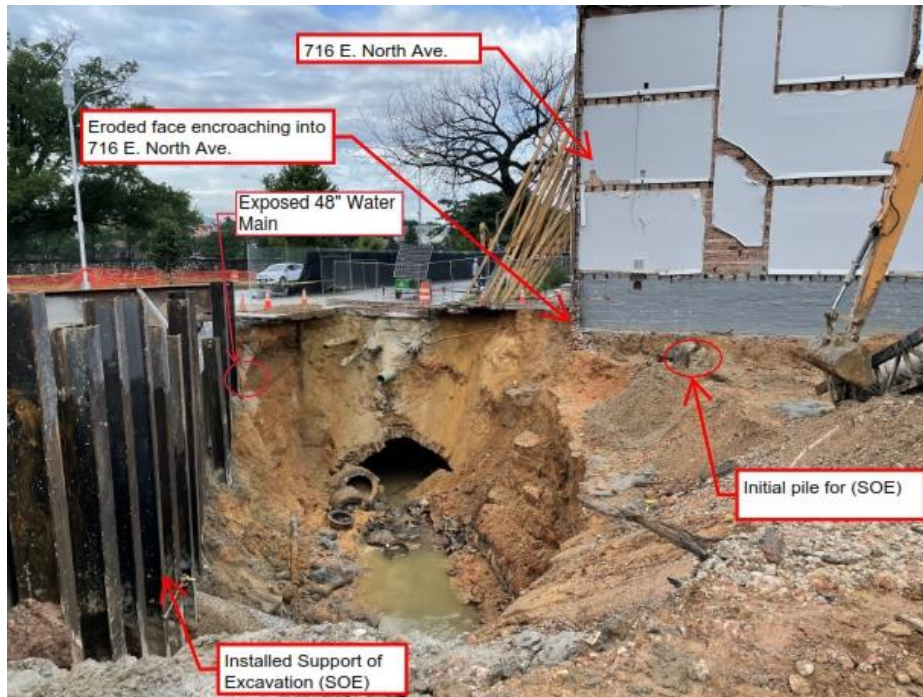
E. North Avenue Storm Drain Collapse August 11, 2022 - 9:31 AM Looking south along eroded storm drain alignment
